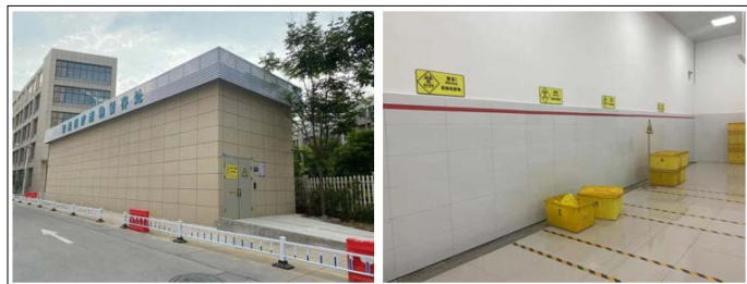
Figure 4: MW Temporary Storage Building Figure 5 Mw Temporary Storage Area
