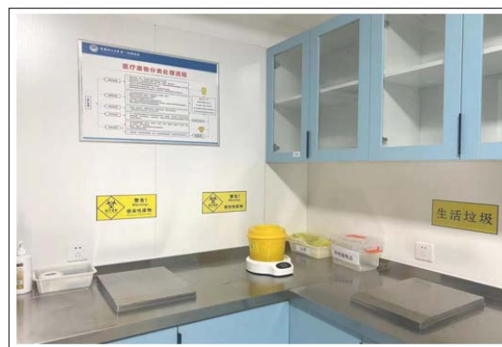
Figure 2: Sorting Table in the Filth Room
