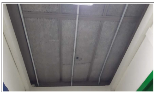
Figure 19: False Ceiling Plate with Asbestos-reinforced Material in a School (author's Photograph)
