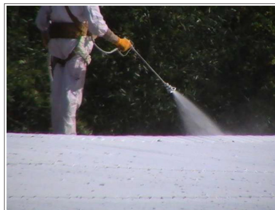
Figure 28: Fiber Fixing Polymer Application over Corrugated Roofing Plate, Prior to Deasbestos Removal. (author's Photograph)
