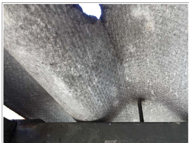
Figure 23: Fiber Cement Plate Fracture. Despite not being a friable material, the deterioration of this material implies the release of fibers and its consequent danger for people who are in the environment, so it is necessary to remove asbestos (author's Photograph)
