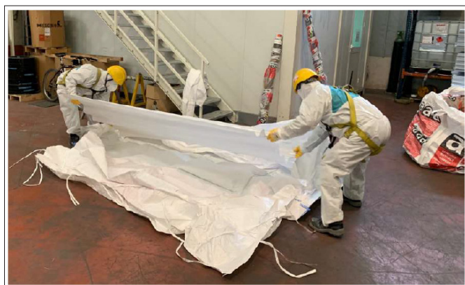
Figure 27: Asbestos Removal Simulation in a Qualification Course for Future Building Roof Removal Operators (author's Photograph)
