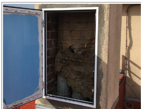
Figure 18: Fiber Cement Chimney Ducts, Protected with Asbestos Sheets for Thermal Insulation, in a Residential Building in Madrid, Spain (author's Photograph).
