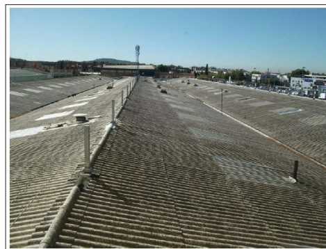
Figure 20: Corrugated Fiber-cement (Asbestos) Sheets Installed in 1970, Forming the Roof of an Industrial Building in Alcalá de Henares, Spain (author's Photograph).
