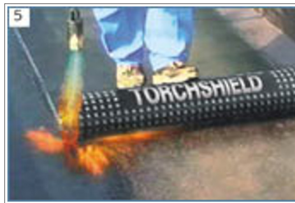
Plate 1: Heat (torch) application of polymer modified bitumen membranes.
