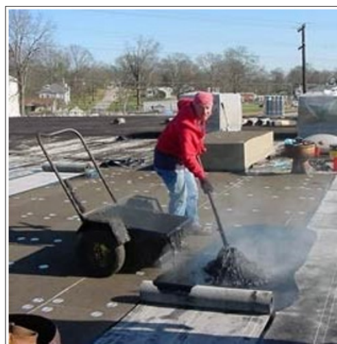
Plate 2: Hot application of polymer modified bitumen membranes.
