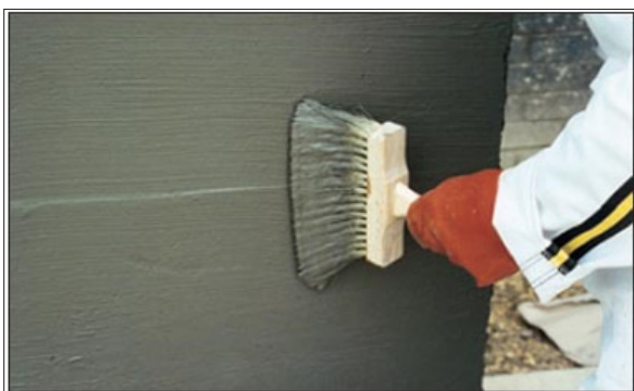
Plate 3: Application of Cementitious Waterproofing Material Source: Arcon supplies, (2017).
