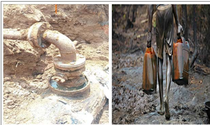
Figure 3: Illegal Bunkering Connection Installed at 12 O' Clock Position on Company Pipeline
