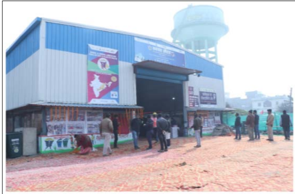
Figure: Bihar, India 1st 10 TPD (Tonne Processing Plant / Day) especially for Dry Waste
